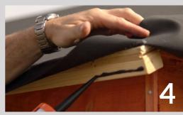
Apply a bead of edge sealant and press the membrane onto it. Once dried this will hold the membrane securely.
