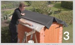
Apply the adhesive working IN STAGES towards the edge of the roof. Roll membrane onto adhesive whilst wet. Re-apply more if necessary.
