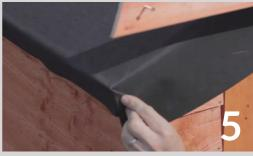
Re-install any existing timber barge boards to help secure the membrane perimeter. Replace if rotten.
