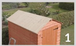
Remove the old roof covering and any nails. Re-board if the roof is rotten or if the roofing felt wont come off cleanly.
