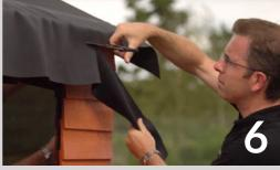
Trim the membrane using a pair of scissors and the underside of the trim as a guide.
