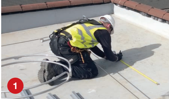
1 Accurately measure and mark out the EJOBAR installation area.
