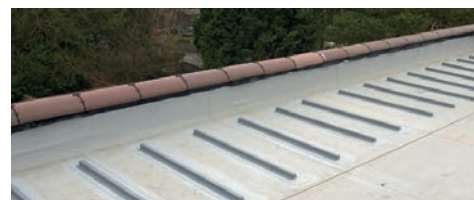
EJObar positioned correctly over membrane strip.
