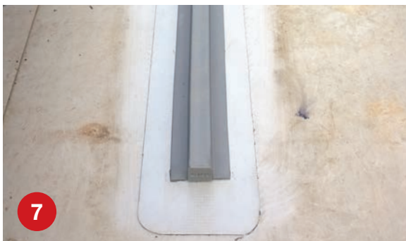
7 How a single EJOBAR looks in position.
