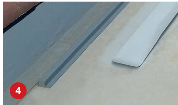
4 Prepare Compatible membrane cover strap, rounding the ends, 100mm longer than the bar.
