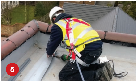
5 Hot-Weld the membrane strap which should be 150mm in width to seal over the fixing line, taking pressure off the existing membrane
