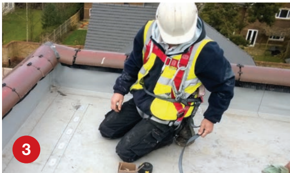
3 Apply correct fasteners for the application at centres determined by a Wind Load Calculation.
