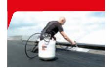
Product application without any need for naked flames is a requirement we have taken into consideration in our application techniques. The HERTALAN® seam joining method is implemented using hot-air technology and an EW joining edge that is readymade in the factory. An emerging welding bead indicates an ideal and permanently safe seam connection. Alternatively, seams can also be adhered together.
