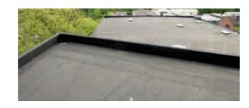
HERTALAN® is a plasticiser free material that is permanently resistant to UV rays, ozone and other natural atmospheric influences and is also extremely elastic within the temperature range of -45°C to +120°C. Thanks to its outstanding elasticity of up to 500%, it can be put to flexible use in various waterproofing situations. HERTALAN® withstands all tensile stresses that a flat roof is exposed to during the course of its normal life cycle.
