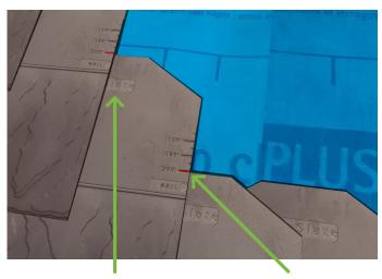
Each slate has embossed guidelines to aid location; the **vertical lines** at the top of the slate assist in locating slates horizontally.
