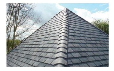
The following instructions are just a guide, and standard roofing procedures should be applied. Installers should follow guidance given in BS5534 – construction of pitched roofs (section 4), BS 5250 moisture management and ventilation and BS 8000-6 workmanship. Eco Slate is impermeable to water so requires the installation of a suitable external membrane over the sarking board.
