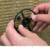
... which is pushed on afterwards as far as the insulation material.
